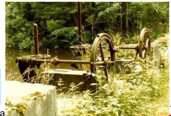
Condition of hydromechanical equipment
